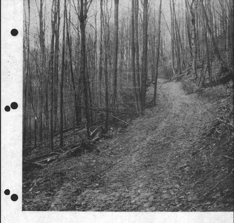
A good skid road like this can be used for future logging jobs. The grade is slight, water is drained off properly, and erosion is kept to a minimum.
