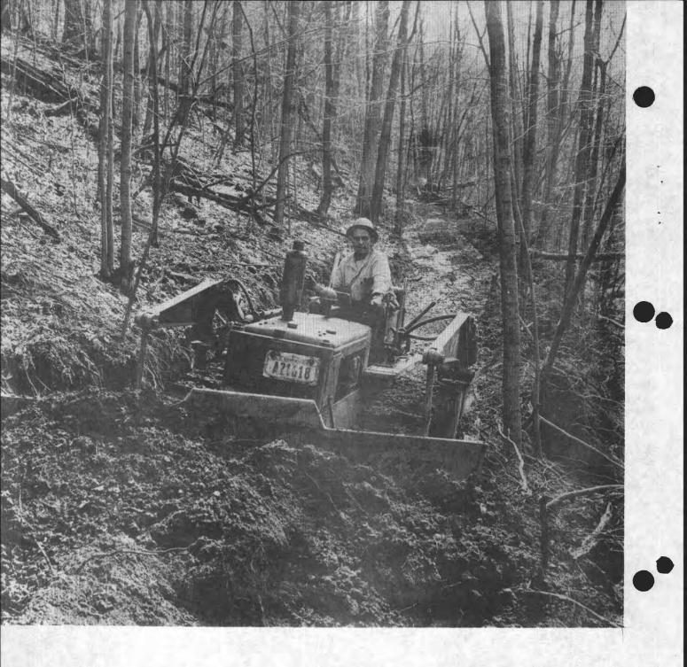
Building a logging truck road. Driving the bulldozer to the top and building the road from the top down is the recommended practice.
