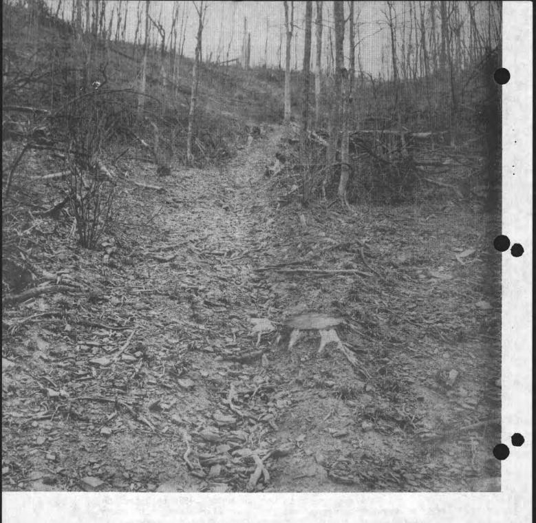
A poor skid road on a steep slope. Already runoff is tearing the road to pieces and ruining the stream below.
